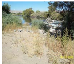
Pre-project, note the raised water level and rock/rubble dam
