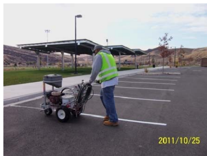
Ryan Thran restriping parking spaces at Golden
