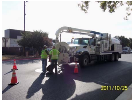
Allan Pagni and Jim Bass cleaning sewer lines on Marietta
