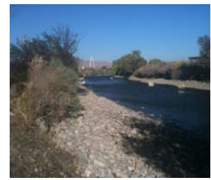
Post-project, note the removal of the dam and restoration of the river to its natural flow
