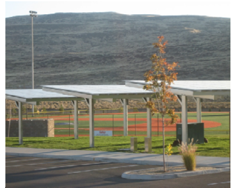
Golden Eagle Park Solar Panels
