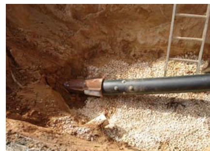
Insertion of the pipe bursting tool into the existing pipe
